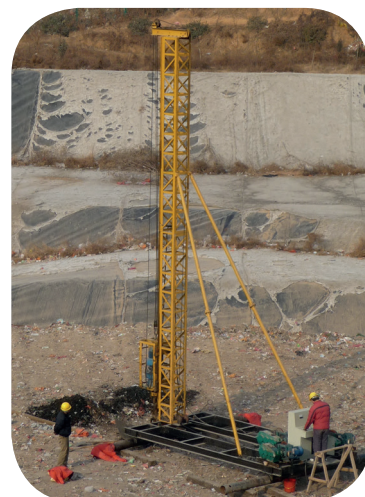
Degassification drilling at Jiyuan landfill site.
